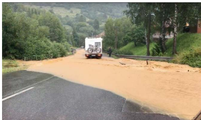
Fig.10: Strong rain undermined the main road that leads through Kremnické Bane.
